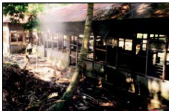
Destruction caused by Tsunami in Nancowry
