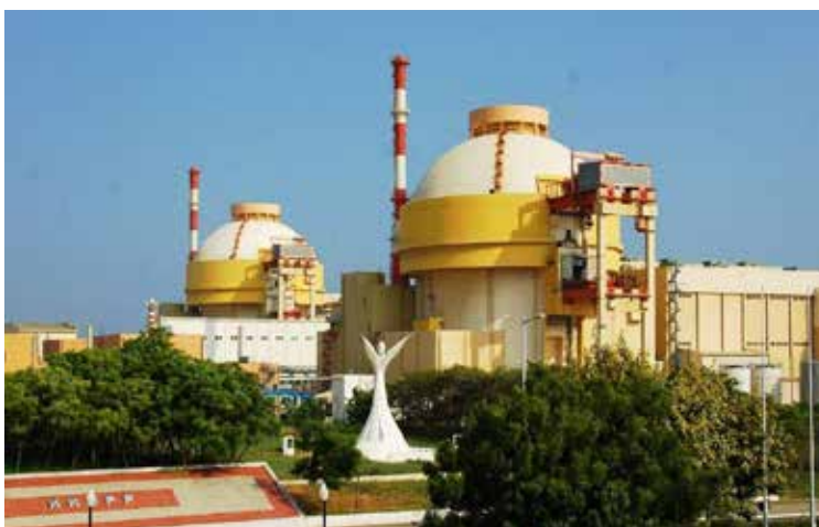
Kudankulam Nuclear Power Plant (KNPP) in Tamil Nadu
