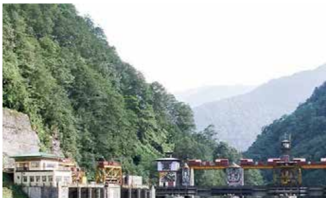
A hydropower plant in Bhutan
