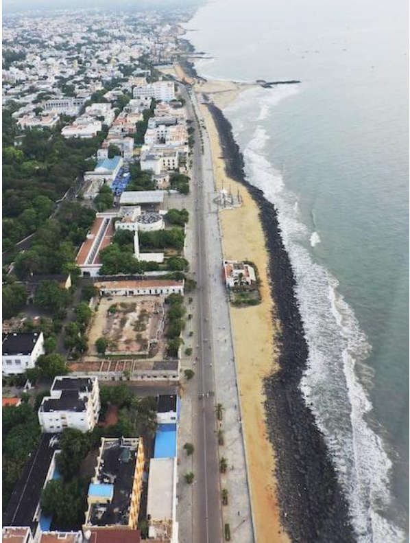
Seawall in Puducherry
