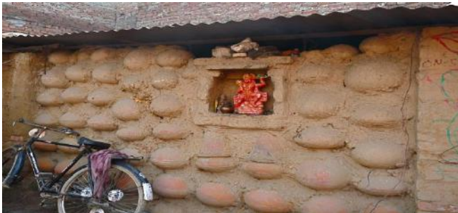
An earthen pots insulation system on a wall in Surat, Gujarat
