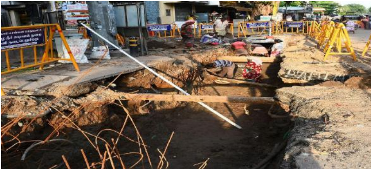
Stormwater drain project in Chennai, Tamil Nadu
