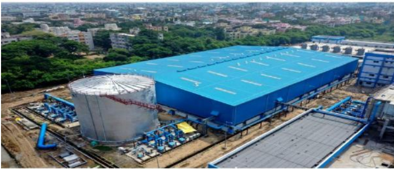
The 45 MLD Tertiary Treatment Reserve Osmosis (TTRO) plant in Chennai
