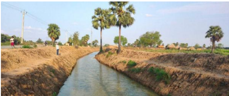
Ahar Pyne floodwater harvesting system in Bihar
