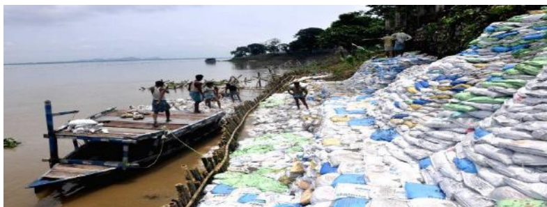
Embankment along the Brahmaputra River in Assam
