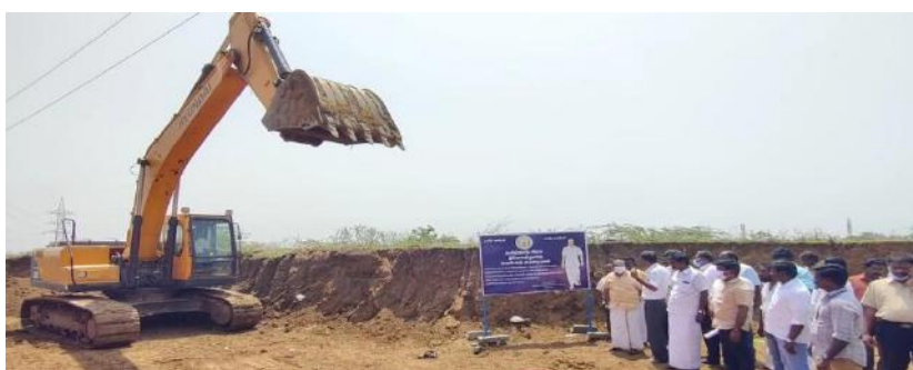
Widening the Adyar River's floodplain in Chennai
