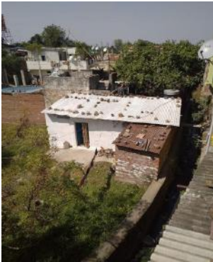
A low income house painted with white colour in Madhya Pradesh
