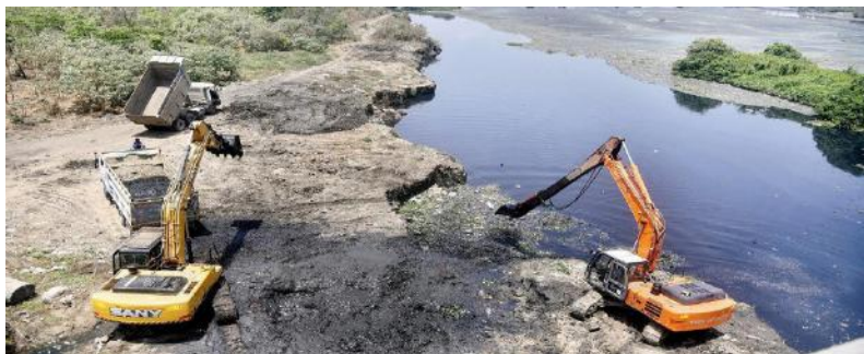
Dredging the Mithi River in Mumbai
