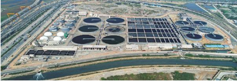
The 318 MLD capacity Coronation Pillar sewage treatment plant in New Delhi
