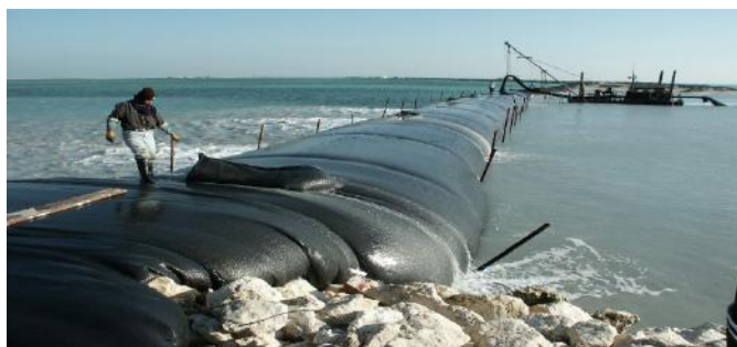
Installing geotextile tube along Odisha's coast
