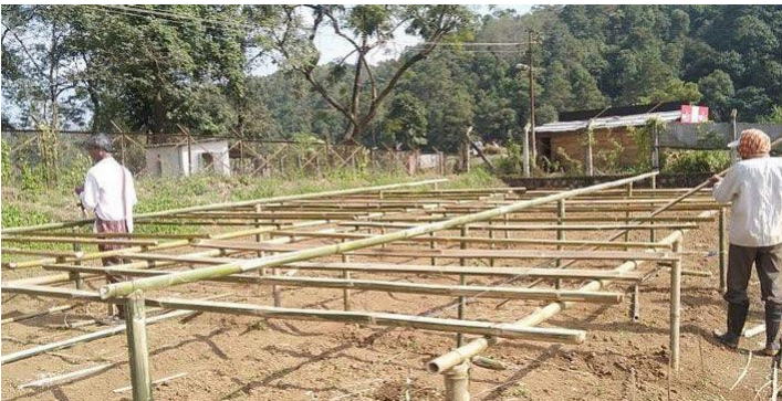
Layout of modified bamboo drip irrigation system in Meghalaya
