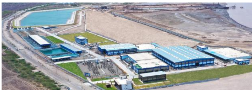
The 100 MLD seawater desalination plant in Debej, Gujarat
