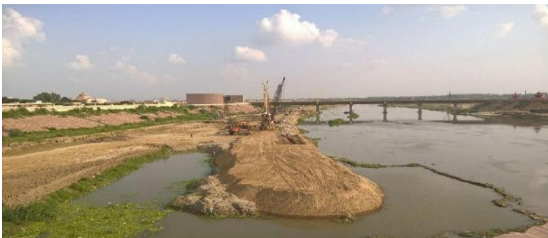
Channelization of the Gomti River in Uttar Pradesh
