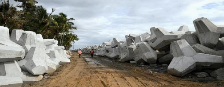
Tetrapod seawall in Kerala
