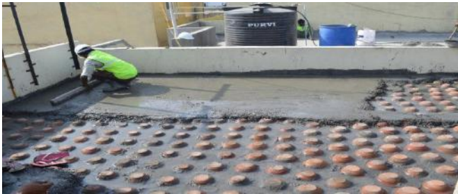
Demonstrating earthen pots insulation system on a roof in Surat, Gujarat
