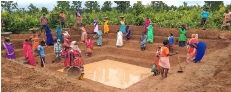
Digging Dobha in Jharkhand
